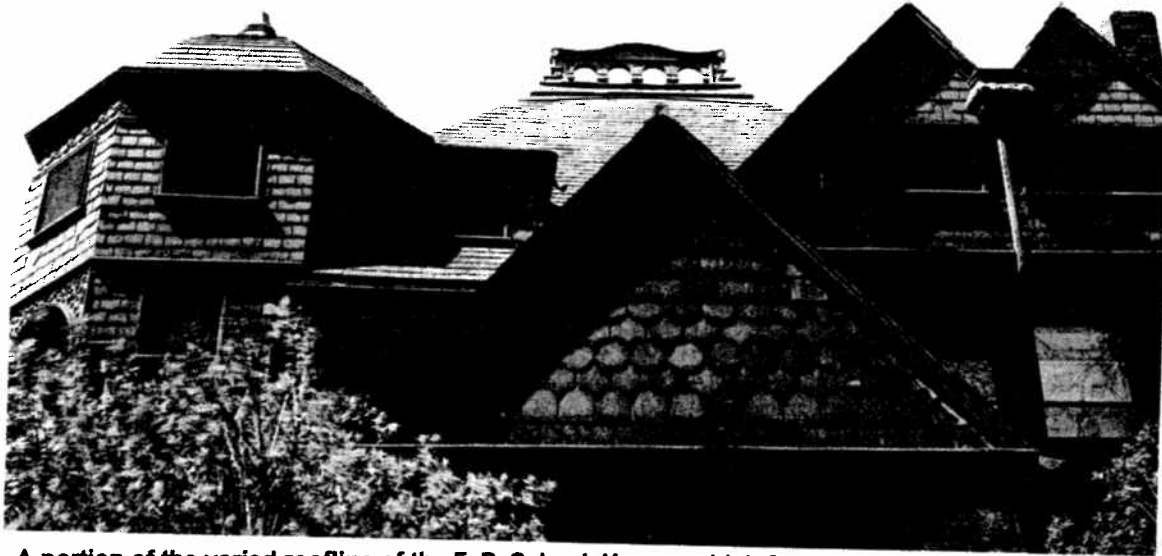
A portion of the varied roofline of the F. R. Schock House, which features a wide variety of details (e.g., "handle" at roof peak) and materials, including slate, pressed metal, and wood shingles.
